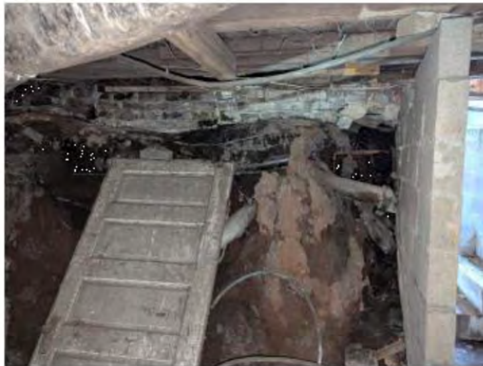
Undermined foundation
