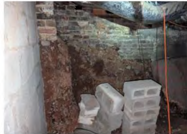
Erosion, failing brick foundation wall, no footing
