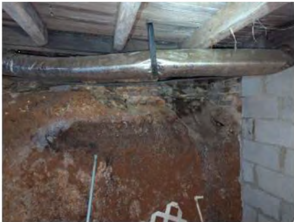
Undermined foundation
