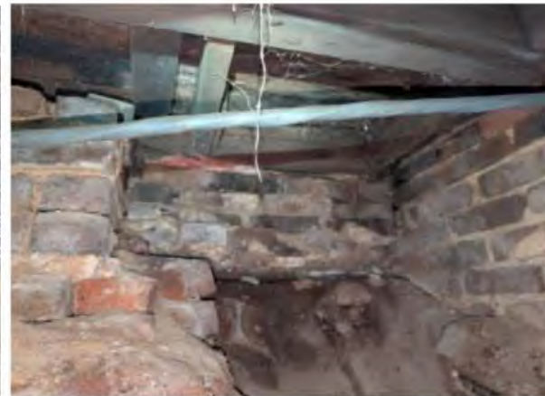
Failing brick wall
