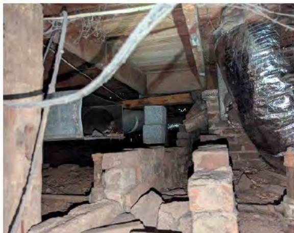
Failing brick, poor supports
