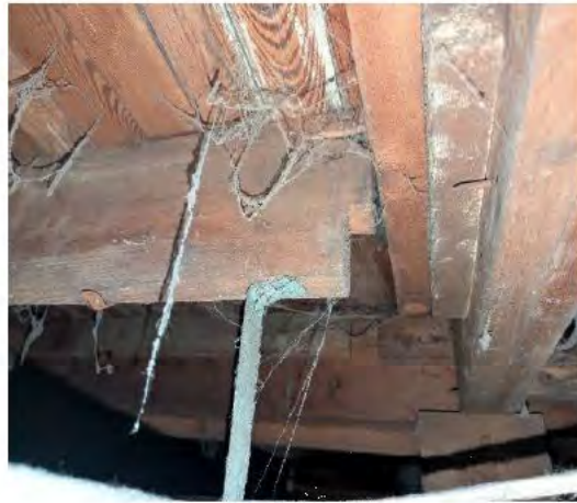
Joists are over notched at girder, pulling away
